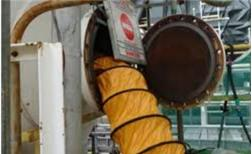
The OSHA standard directs that, before an employee enters the space, the internal atmosphere shall be tested with a calibrated direct-reading instrument for the following conditions, in the order given: 1) oxygen content, 2) flammable gases and vapors, and 3) potential toxic air contaminants.
