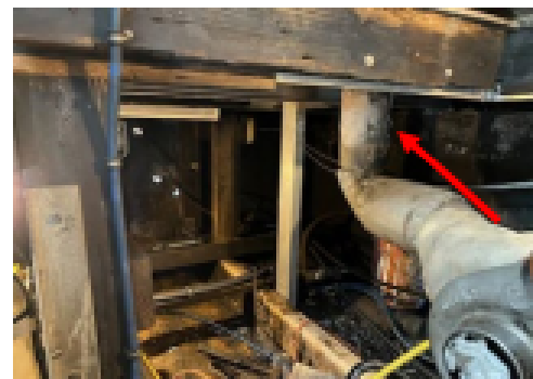
Dry exhaust passing through wood/FRP deck
