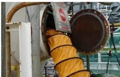
The OSHA standard directs that, before an employee enters the space, the internal atmosphere shall be tested with a calibrated direct-reading instrument for the following conditions, in the order given: 1) oxygen content, 2) flammable gases and vapors, and 3) potential toxic air contaminants.
