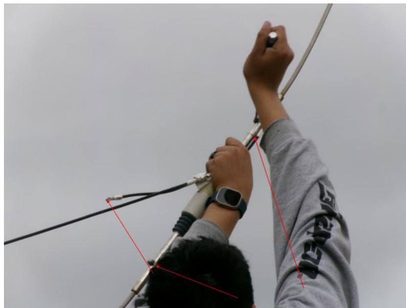
Jumper wire connected across the insulator removed from the clip here.
