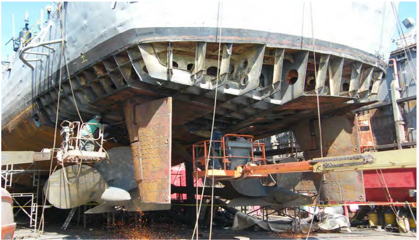
U.S.S. LAFFEY (DD-724) receiving new 3/8" hull plating from bow to stern, port to starboard to 1' above existing waterline. Vessel was drydocked on AFDL-47 for the entire restoration.
