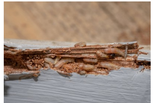
Wood Termite Frass (poop) Dry Wood Termite Infested Wood (larvae and frass)
