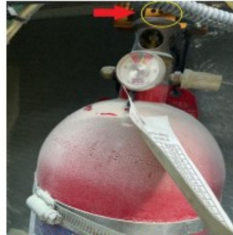
Figure 4 Sea-Fire NFD 500 Series safety pin placement
